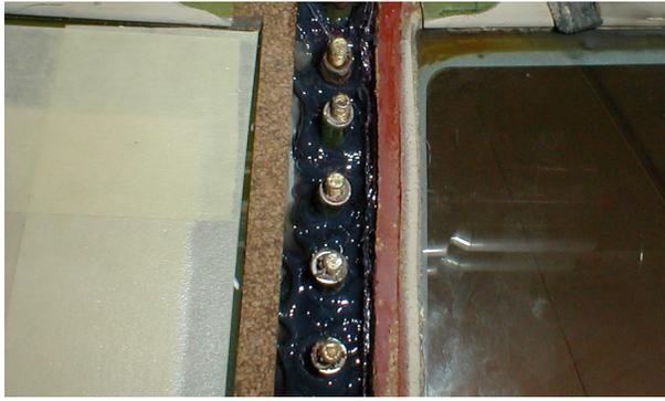
Thixflex Black® installed in panel to create water tight seal
