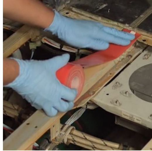
HI-TAK Polyurethane Rolled Sealant Installation
