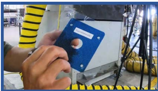
Antenna Gasket Installation
