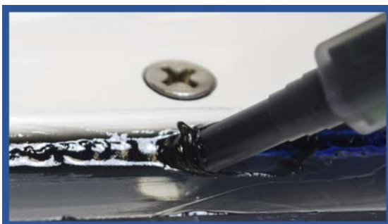
Injectible Sealant Priming & Installation
